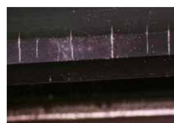
Heat aging Material fracture and hardening from exposure to temperature beyond material limits.
