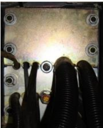
Feed Thru's installed
