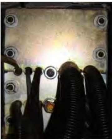
Feed Thru's installed
