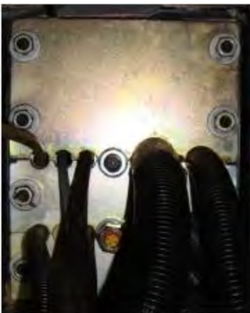
Feed Thru's installed
